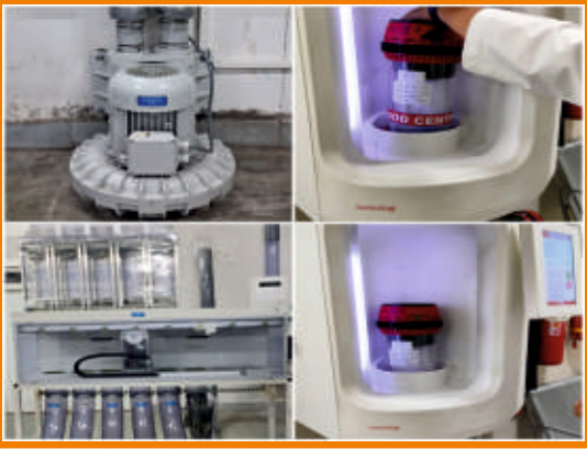
Figure 1 Parts of pneumatic tube system: [a] Blower [b] pneumatic tube system carrier with blood bag and receiving basket [c] Polyvinylchloride tubes [d] leak proof pts carrier with cushion with attached computer screen.
